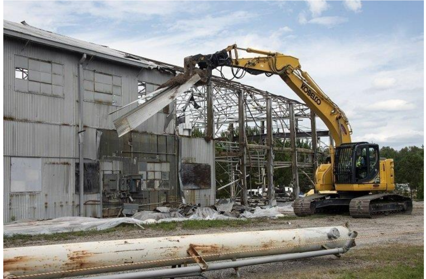
Workers demolish a section of the metal roof over the Ford Building at the Savannah River Site. At the height of the Cold War, the facility was used to test components used in five nuclear reactors at the site.
